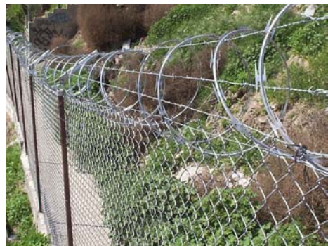
The new chain link fence surrounding La Roca.
